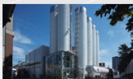
Silo and discharge systems
